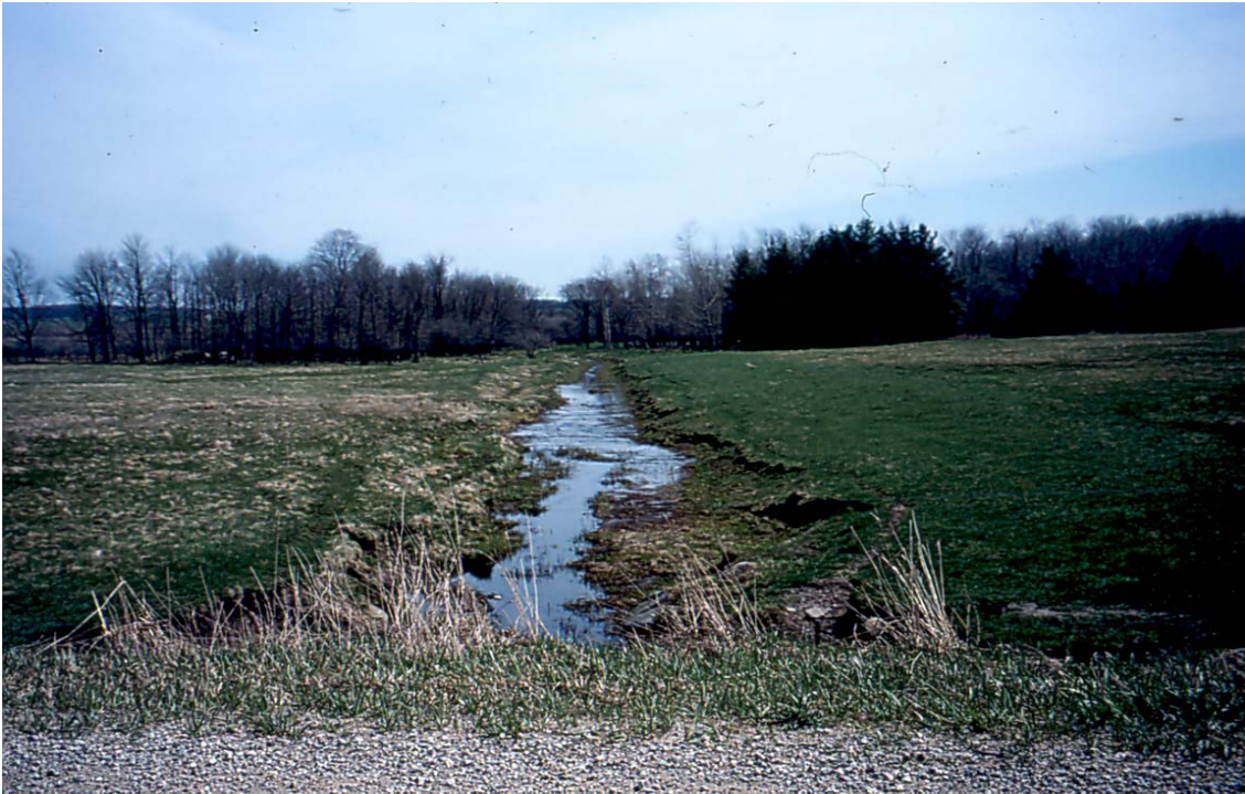
Fig. 2: Campbell Drain tributary, pre-restoration 2001 (Source: GRCA).
